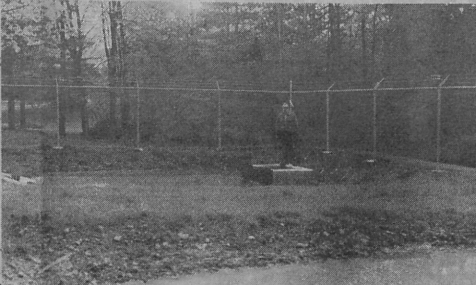
Settling basins for dirt and filtered water. Water runs from here to sewage treatment plant and on through to canal.
